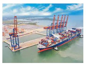
Gemalink deep-sea port is one of the seaports with the deepest draft in Vietnam, and with this specification, Gemalink port is one of the few seaports has a strong attraction to shipping lines, especially those operating mother vessels with a tonnage of up to 250,000DWT – the world's largest container vessel size to optimize operational efficiency nowadays.
